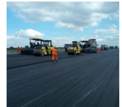
Works on modernization and expansion of the airport
